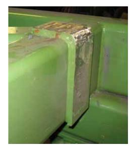
3) After removing the upper cylinder ear, torch off the existing lollipop weldment located on the wing running gear leg, while again leaving the base plate intact. After torching, grind the base plate surface flat so it is suitable for welding.
